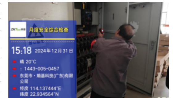
▶ Monthly Comprehensive Safety Inspection
